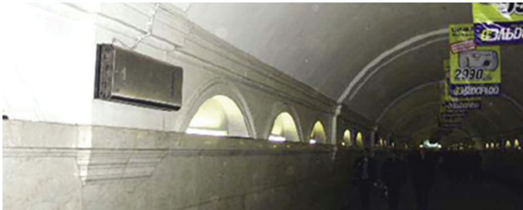
Recirculator AR-UF-170-2 mounted in the passage between “Paveletskaya-Radial’naya” and PaveletskayaKoltsevaya”
